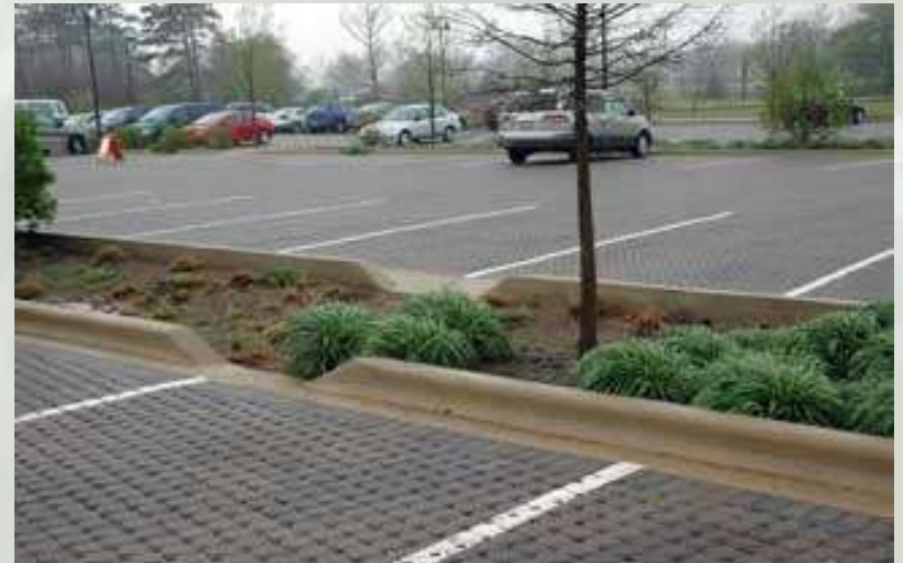
Permeable paver parking lot
